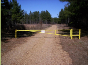
Blocking public access. KC Zoning Code Violation § 19.02.060
